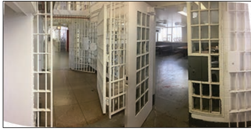
DETENTION RM ENTRANCE
